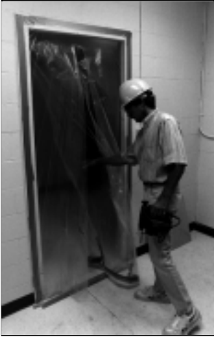
Close off entryways with an airlock.
